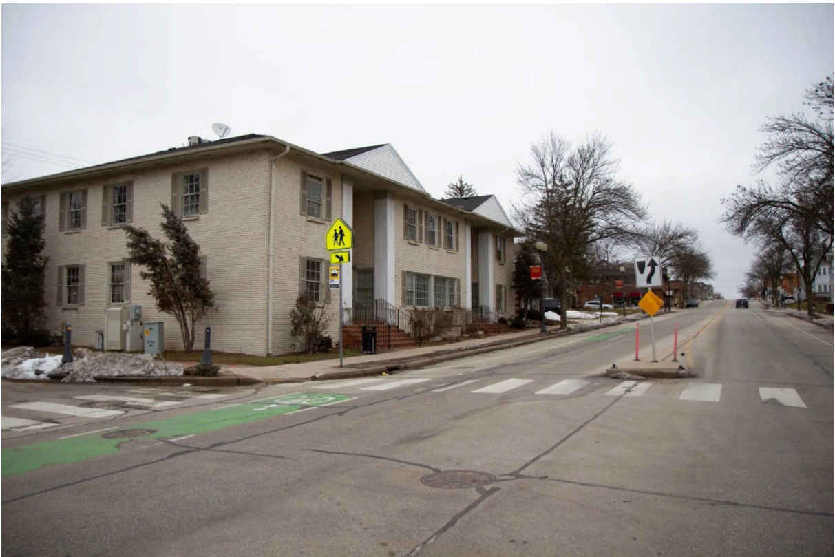
THE IDYLL BUILDING BEFORE RENOVATION · 6330 W. NORTH AVENUE, WAUWATOSA
